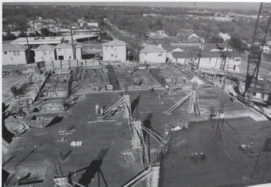
A growing campus. Construction of the six-story Health Science Education Building on the UNT Health Science Center campus is going well. Here, workers pour the floor and build support columns for the first floor. An addition to Medical Education Building 2 is at the half-way point in construction.
